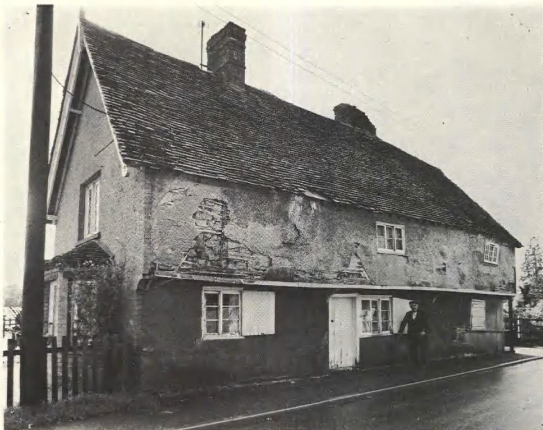
Plate 1 'Rowe's Cottage', Little Barford, before stripping. Photograph: Bedfordshire County Council.
