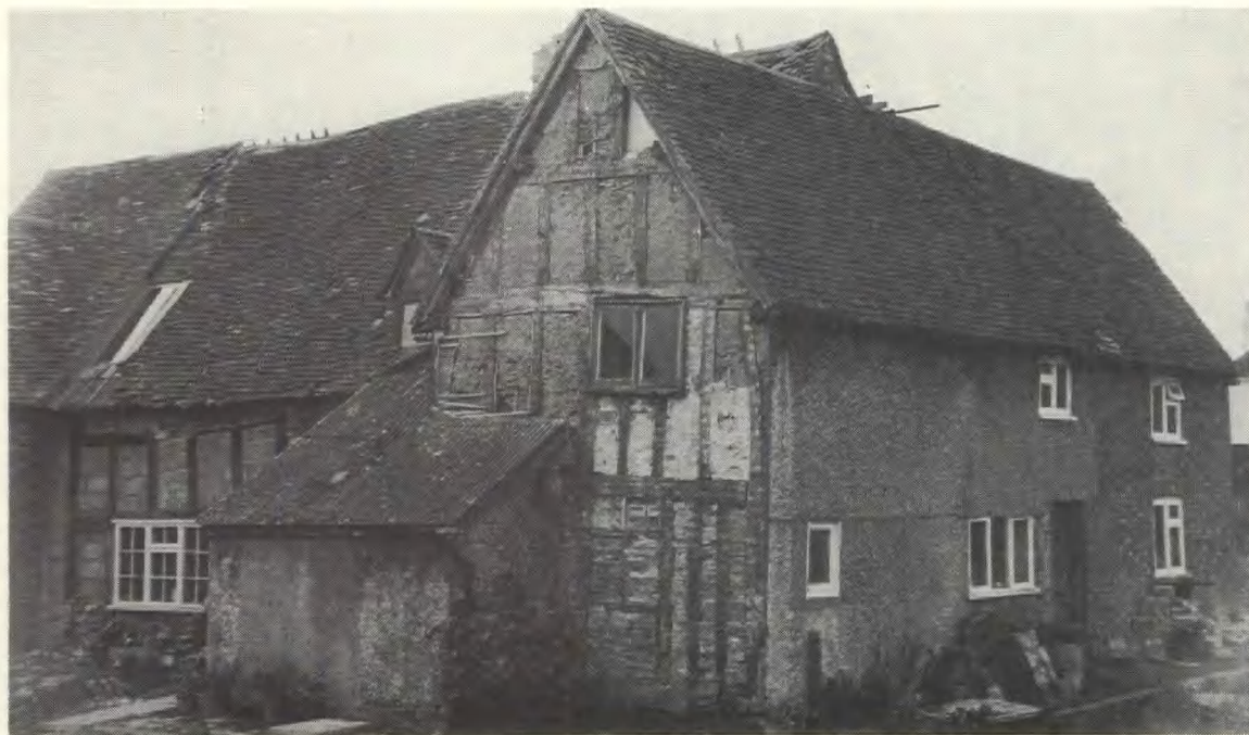
Plate 1 Lower Roxhill Farm, Marston Moretaine: from east.
